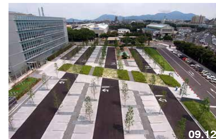
Figura 09.12. e 09.13. NSE Kitakyushu Technology Center, Fukuoka (Giappone). PLATdesign. [Fonte: http://landezine.com/index.php/2013/01/nse-kitakyushu-technology-center-by-platdesign/ ] Figura 09.14. University of Applied Sciences Ruhr-West in Bottrop, Bottrop (Germania). Planergruppe Oberhausen. [Fonte: http://landezine.com/index.php/2018/12/university-of-applied-sciences-ruhr-west-in-bottrop-by-planergruppe-oberhausen/ ]
